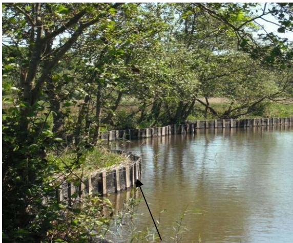
Original design timber posts replaced with recycled timber piles
