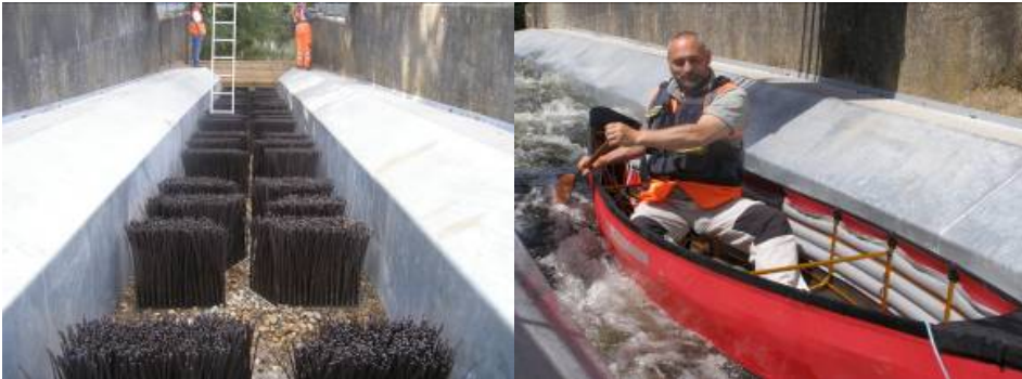
Figure 8. River Medway fish and canoe pass
