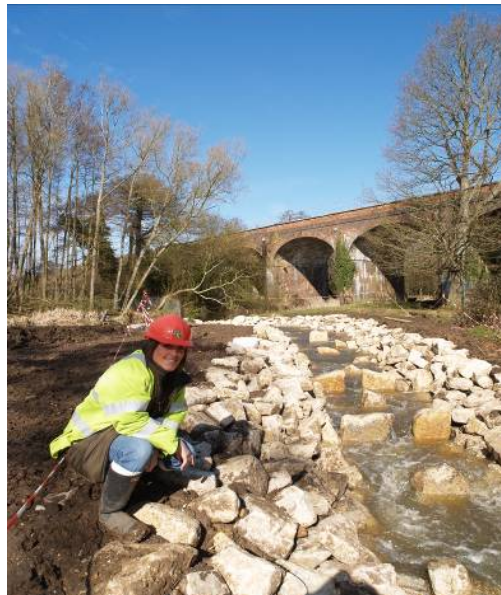
Figure 4. We have improved fish passage at Botley Mill on the River Hamble.
