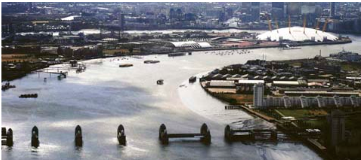
The Thames Barrier has remained a constant feature in the rapidly changing urban landscape over the past 25 years
