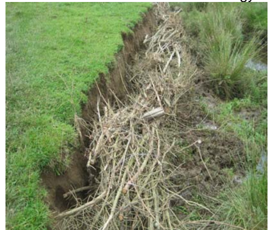
Brash bundles protecting eroded banks.
