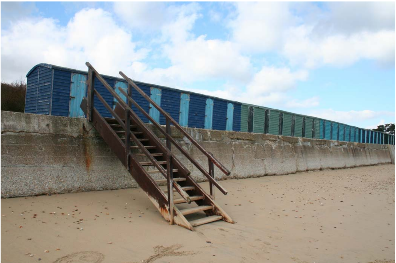
The sea wall on the Duver
