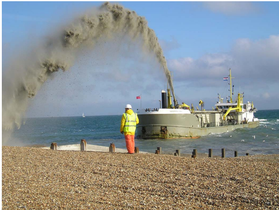
Plate 1 Sospan Dau “rainbowing” shingle onto the beach at Hayling Island (Photograph by courtesy of Westminster Dredging Ltd)
