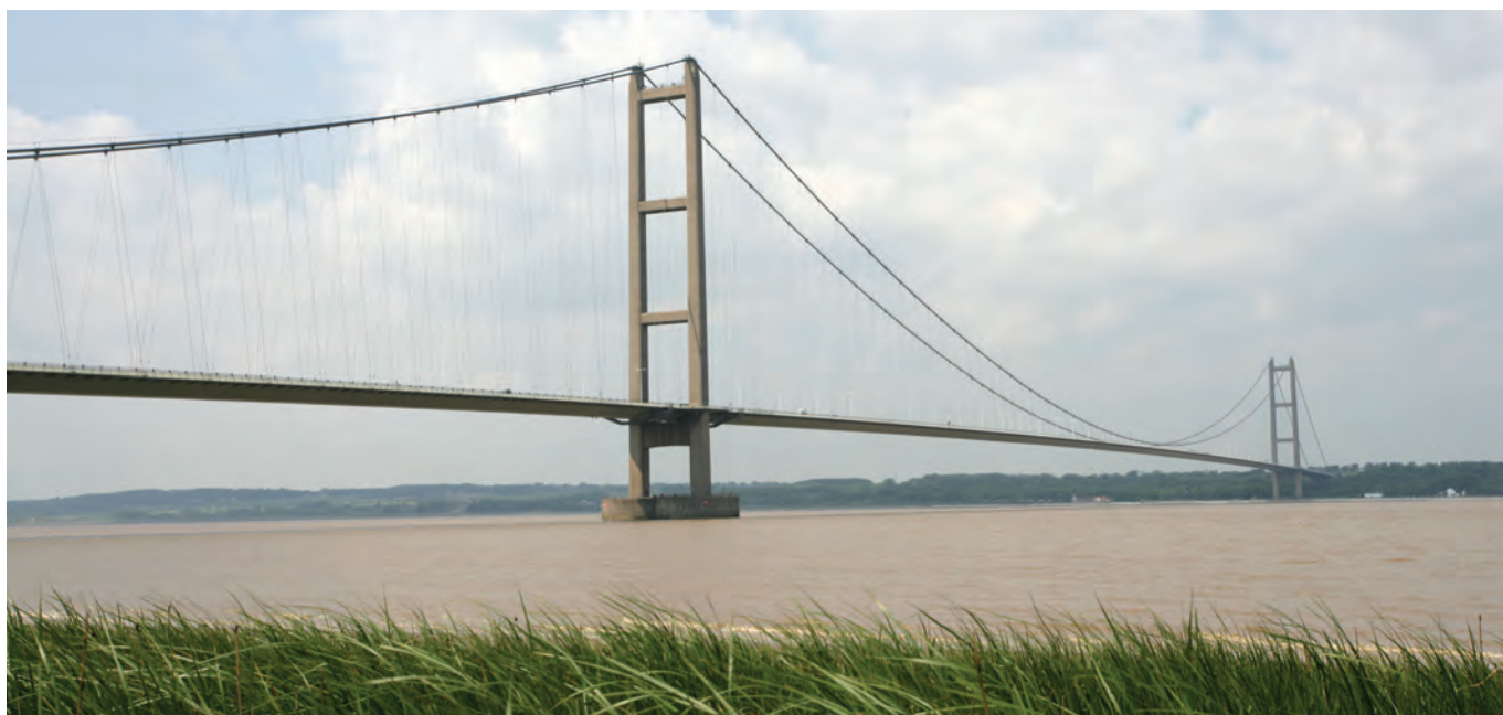
Humber Bridge over the Humber Estuary
